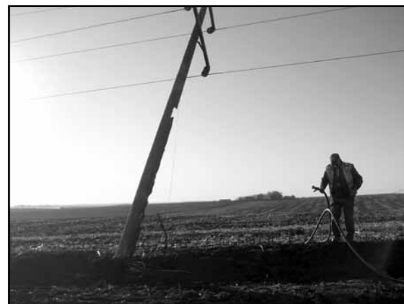
A fireman holds a water hose after extinguishing a pole fire near Newkirk in Sioux County. The pole had to be replaced.
