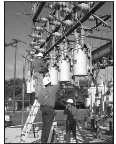
NWREC personnel help NIPCO employees install substitution equipment
