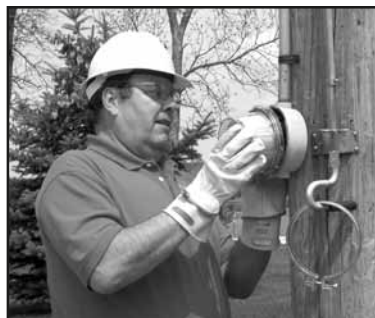
Denny Perry, Member Service Advisor, installing a new AMR meter in Ida County
